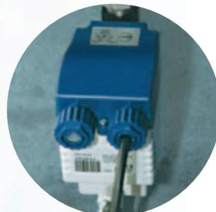
*Electronic level controlled zero loss condensate drain (L120SR).*
