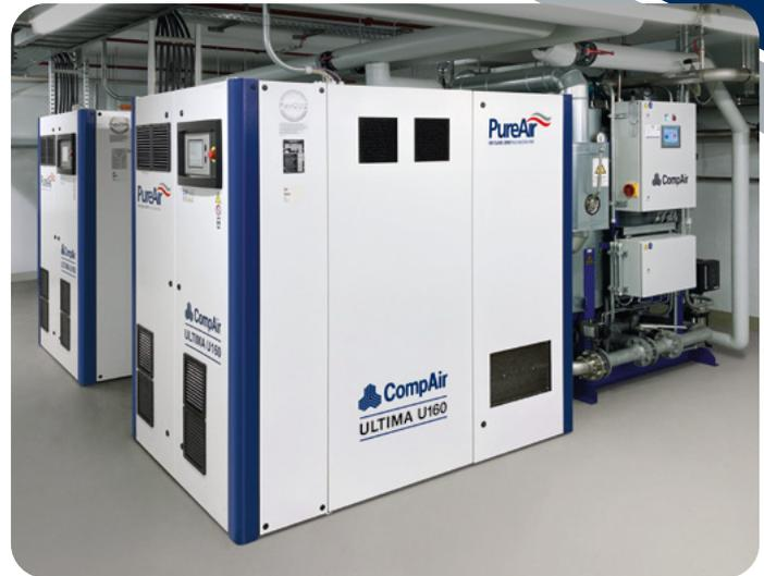
Despite the limited space in the equipment room, two Ultima compressors combined with two HOC adsorption dryers could be installed thanks to the small size.
