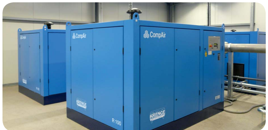
Four identical piston compressors generate compressed air for Wergona – efficiently, oil-free and across eight volumetric flow ranges.
