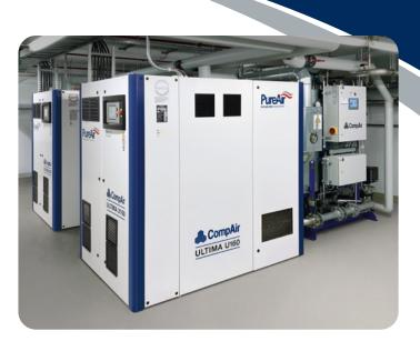
Despite the limited space in the equipment room, two Ultima compressors combined with two HOC adsorption dryers could be installed thanks to the small size.
