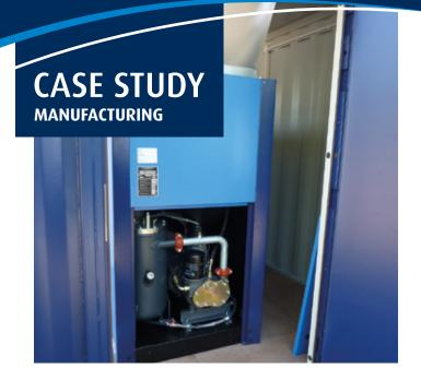
The key issue was that the compressor housing had been constructed around the machine. As a result, it would not be able to accommodate a new system without extensive structural work.
